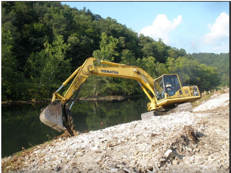
ERS remove vegetation and debris from the river bank.
