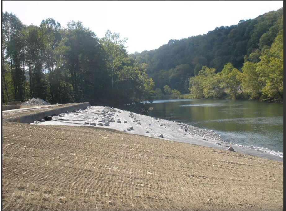
River bank of the Site, covered with geotextile fabric and backfill.
