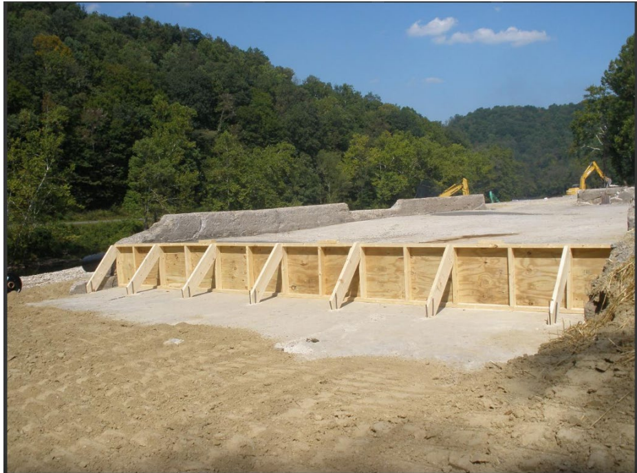
ERRS encapsulate exposed lead-contaminated materials.
