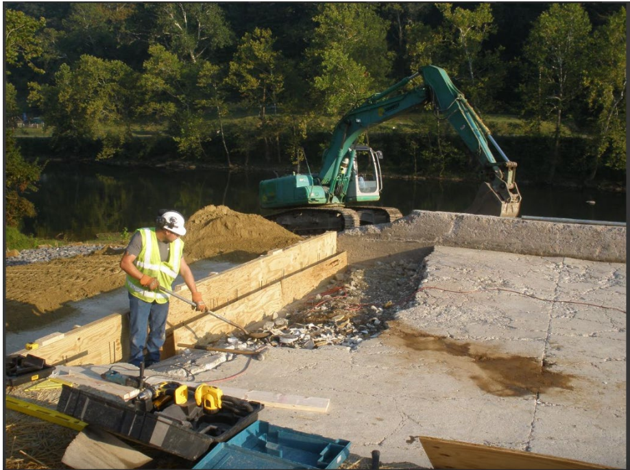
ERRS encapsulate the remaining exposed lead-contaminated materials with concrete.
